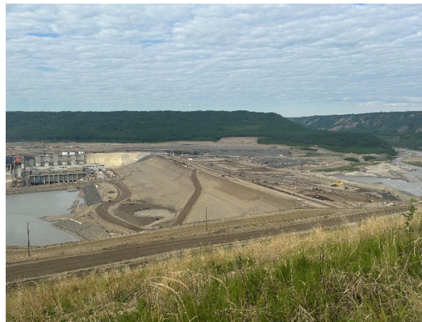
Figure 7: View of the earthfill dam at Site C, July 2023.
