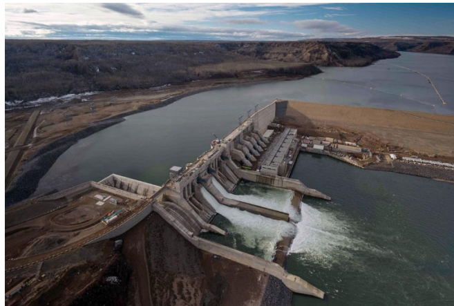
Figure 6: Dam site at Site C, November 6, 2024.
